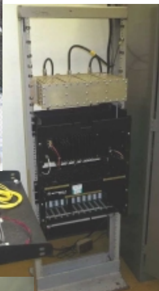
Site visit results: Found DC power supply for port 3 radio was dead. Replaced with original DC supply (fixed by Lorne) Removed TX channel element and cleaned up IDC pot Re-adjusted IDC to spec and rechecked TX deviation on Port 1. Next visit Port 3 radio will be programmed for active high COS along with RLC controller. 73, Lorne & Brad
