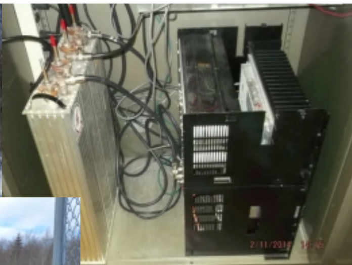
Here are some pictures Lorne & I took today at the Lynn Mtn. site (VE1SPR). We lost our link to Gore and had to replace a power supply. The audio on the VHF Repeater was bassi so Lorne removed the crystal element cleaned the pot and replaced and tweaked it with the IFR, Everything sounded great when we left. Thanks Tom & Shirley for supplying us with the Site Key. Weather was great. Brad VE1ZX.
